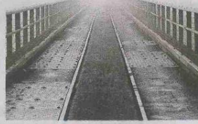
Work will begin on the Peketahi Bridge before Christmas.
